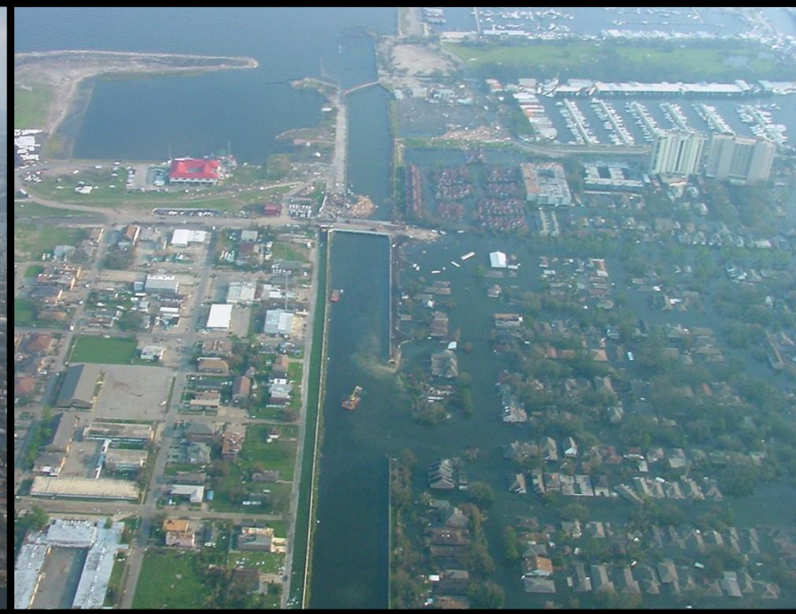
Lakeview Neighborhood, 17 th Canal Levee breach
