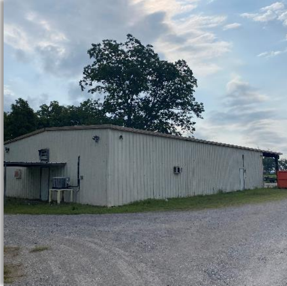
Building 2, Viewed Easterly
